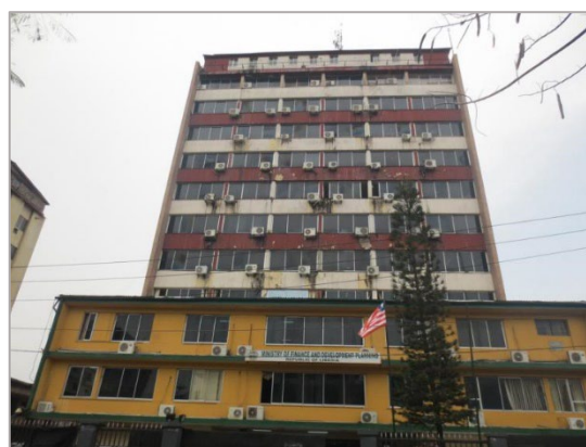
Figure 1: The Ministry of Finance and Development Planning, Monrovia.
